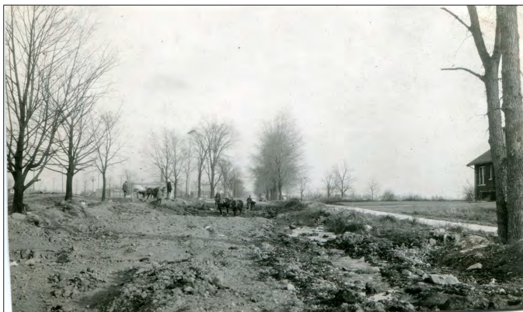
Figure 15. 12 Mile Road looking east from Vinsetta Boulevard showing workmen preparing to excavate for the Grand Trunk viaduct (ROHS ca. 1929)
