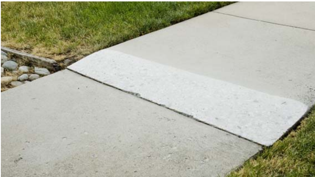
Sidewalk that has had a one-inch differential ground down
