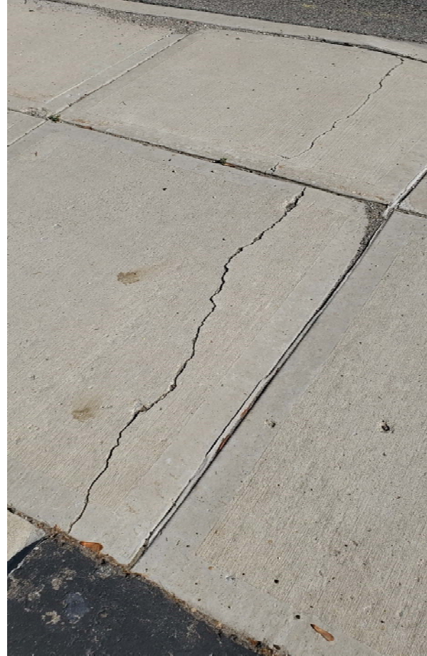
Poorly seated crack > one quarter inch
