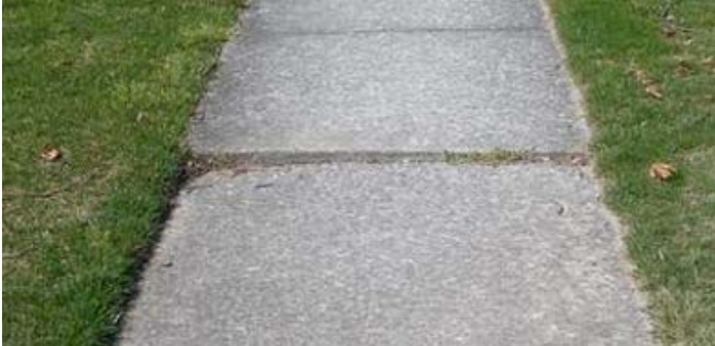
Sidewalk differential greater than one inch
