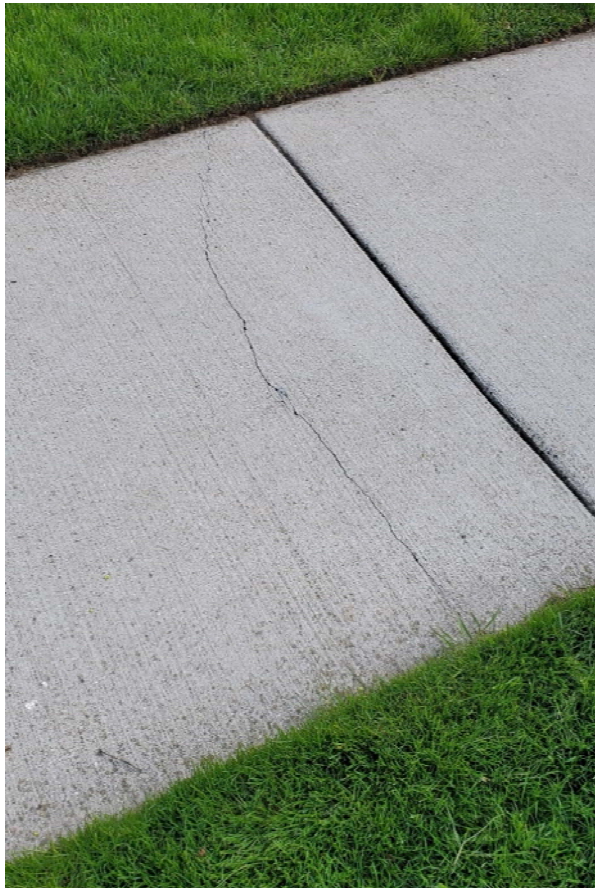
Tight hairline crack with just two pieces
