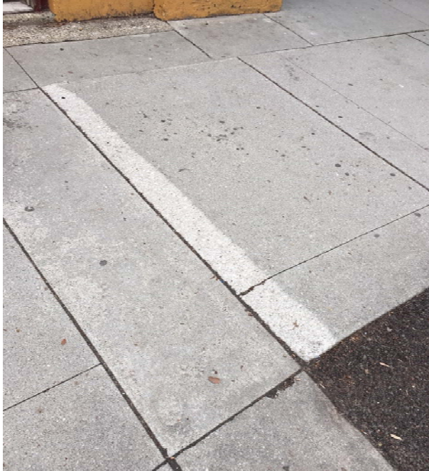
Sidewalk with a three quarters inch differential ground down
