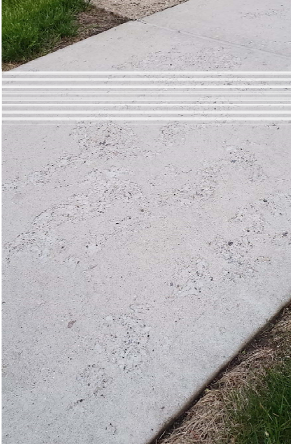
Scaled sidewalk slab
