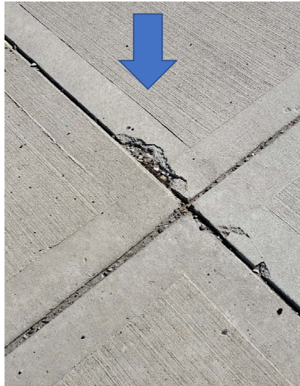
Spalling joint
