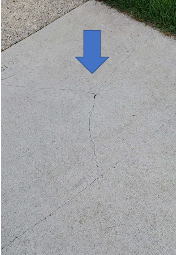
Tight hairline crack however with multiple pieces
