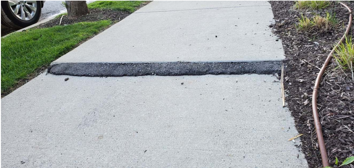
Sidewalk differential greater than one inch, wedged with temporary cold patch, lifted by tree roots
