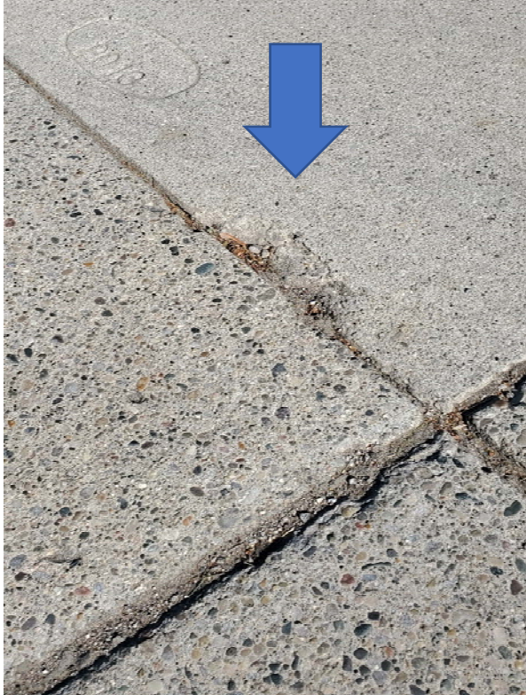
Chipped/deteriorating joint
