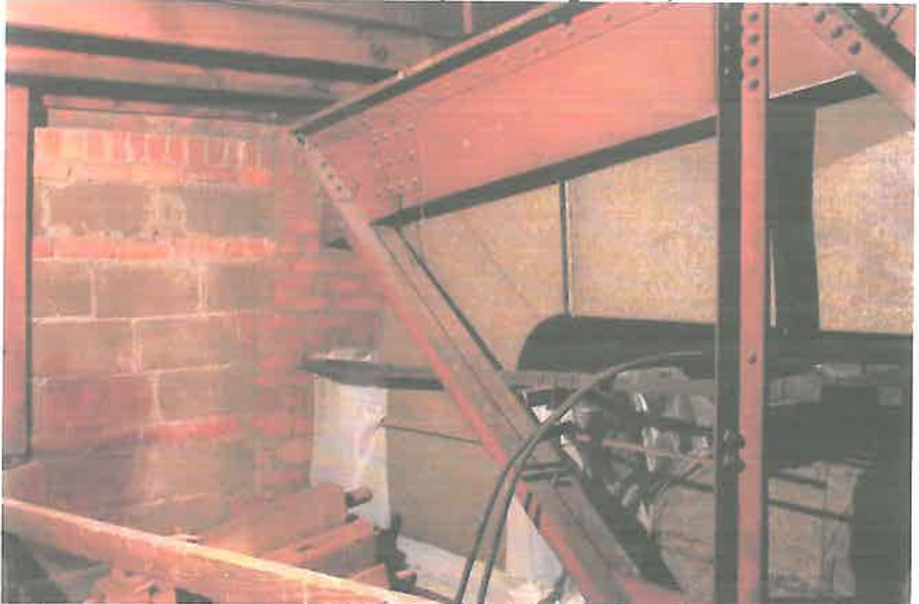
(Attic photo showing masonry bearing walls, steel girder, and wood roof joists)
