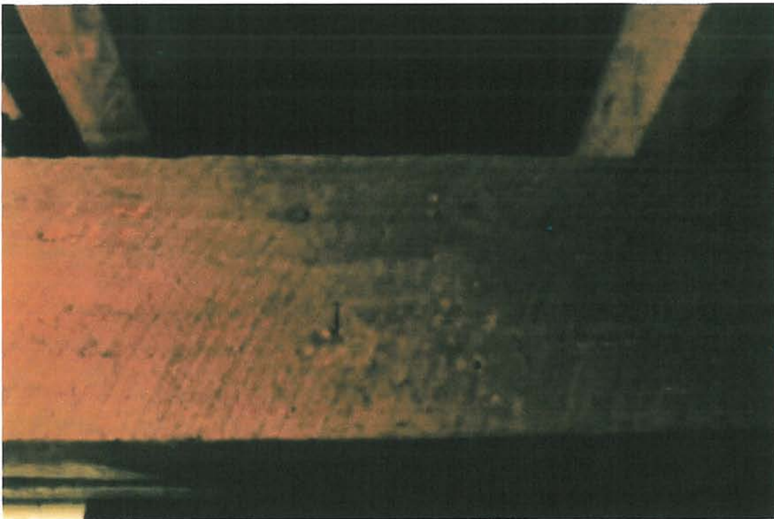
Circular rough sawn first floor joist
