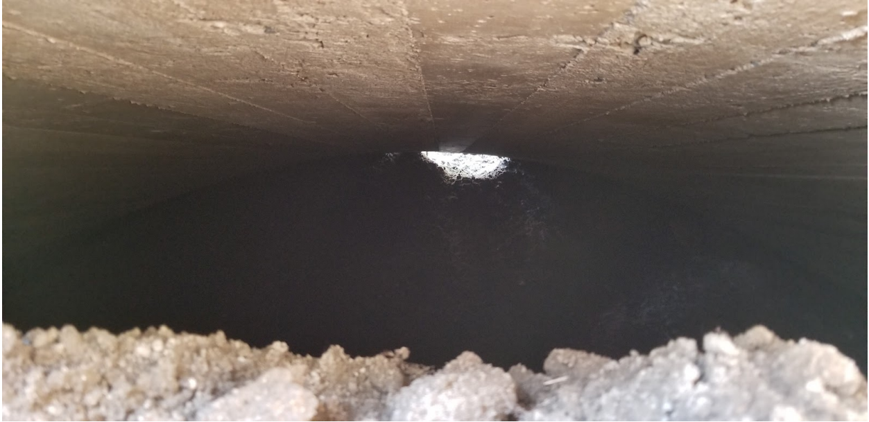
View under and through the Cedar Hill bridge, June 16, 2022. The distance from the bridge road bed to pipe that contains the Red Run is approximately 3-4'. The arch of the bridge to carry traffic over the river is still intact and functions. The original span is still present.
