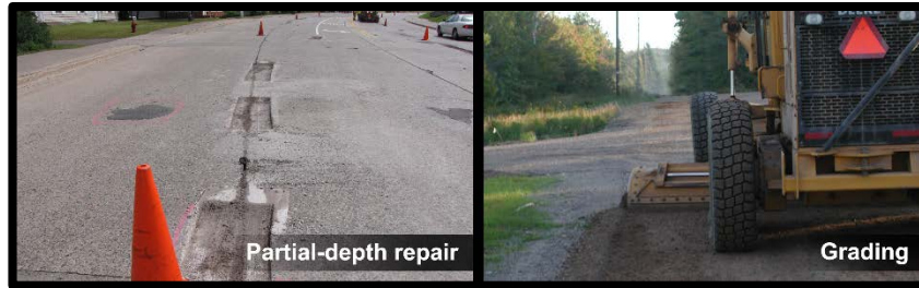
Figure 6: Examples of capital preventive maintenance treatments, cont'd—(from left) concrete road prepared for partial-depth repair, and gravel road undergoing maintenance grading,
